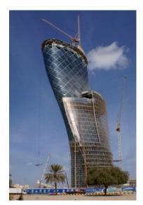
The core was built using formwork resettable technology. Firstly it is made a dense grid of steel rebar. Then around it is set the formwork in the form of the core; steel grid is poured by concrete. Then it is possible to rise up the formwork and repeat the same operation. As concrete will fill 4 meters there are set a few bars and the formwork is raised to the next level with the help of hydraulics. [1]
