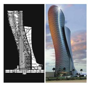
The tower rising out of the ground at 160 meters forms the angle of 18° with the vertical axis. The difficulties of this project begin on the first day. Upper floors are outside of the foundation line at 33 meters. Because of this appear a huge forces, which aimed to pull the foundation of the building out of the ground. The work begins with the foundation, located deep underground. [1]
