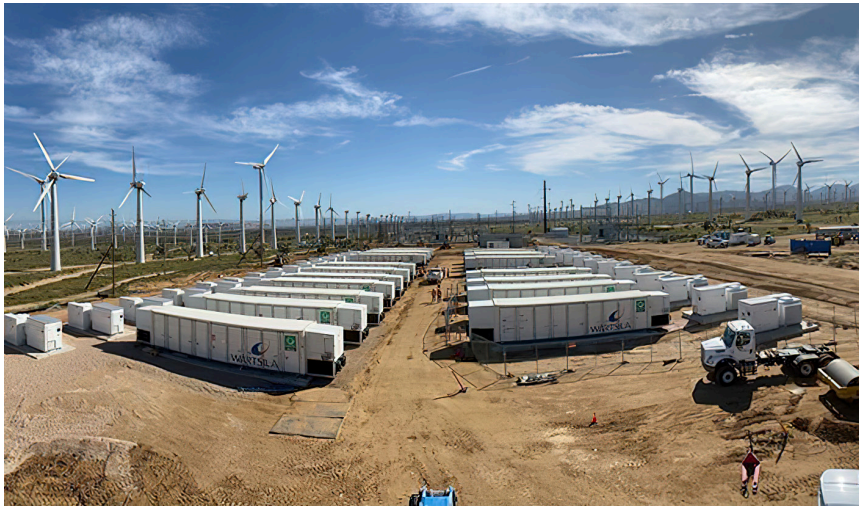
Рис. 2. Gateway Energy Storage [5]
