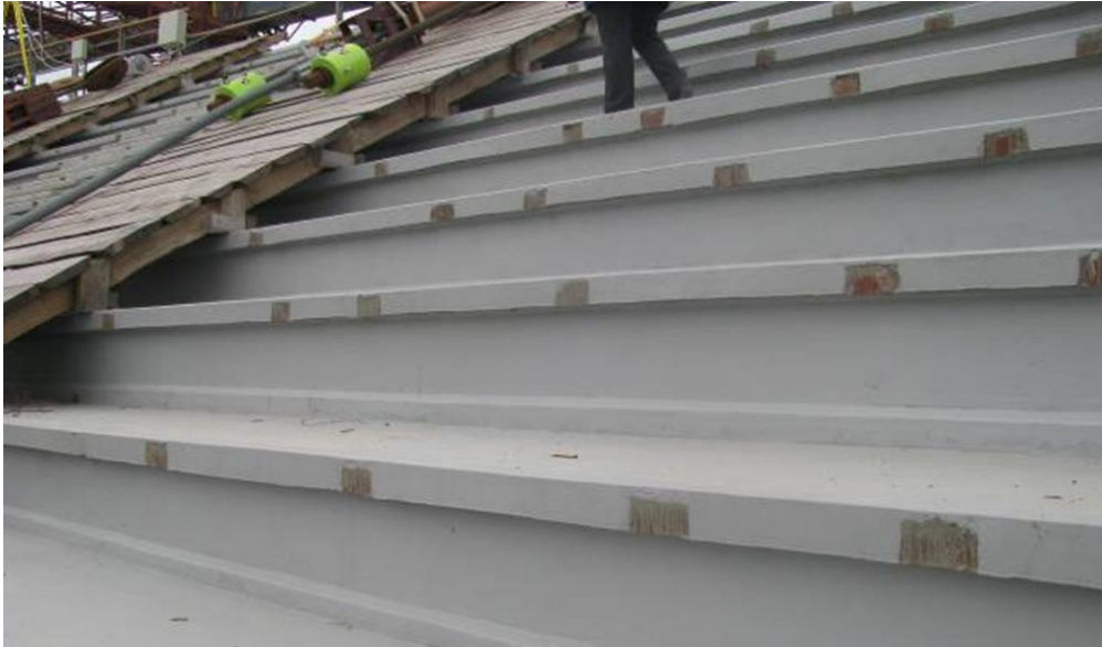
Fig.3. Folding panel appearance after finishing repair and restoration works
