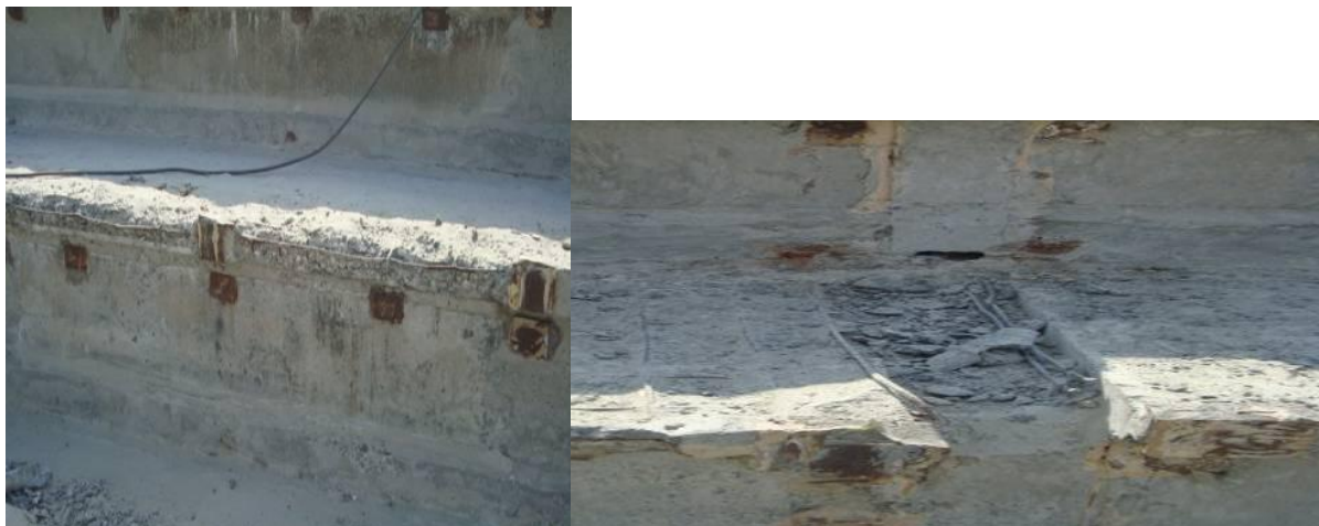
Fig.1.Reinforced concrete construction damages of folding panels after cutting off encrustation from concrete repair mortars
