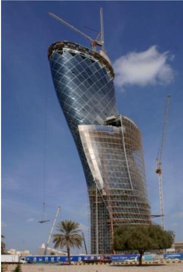
The core was built using formwork resettable technology. Firstly it is made a dense grid of steel rebar. Then around it is set the formwork in the form of the core; steel grid is poured by concrete. Then it is possible to rise up the formwork and repeat the same operation. As concrete will fill 4 meters there are set a few bars and the formwork is raised to the next level with the help of hydraulics. [1]
